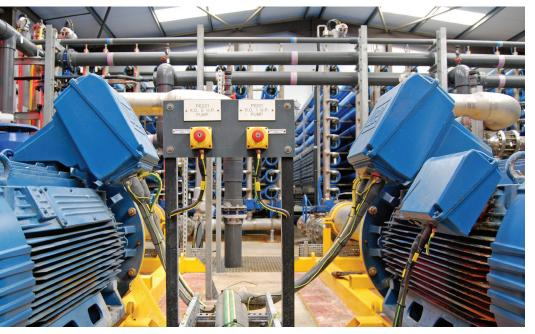
The upgrade involved the installation of a large number of new pumps, almost all of which would need to be controlled by
